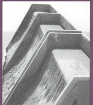
Wastewater Treatment For Roofing Manufacturer
